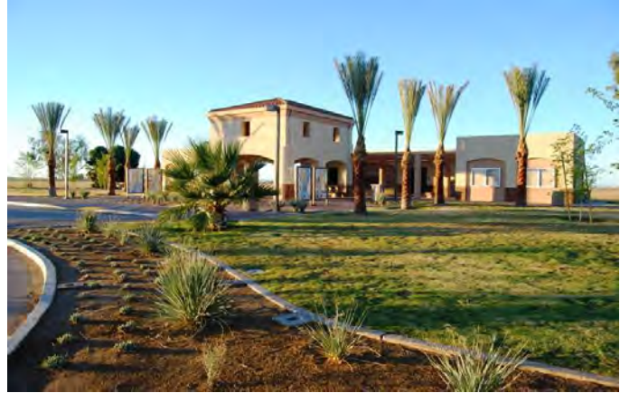
Sunbeam Rest Area on Interstate 8
