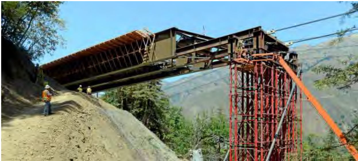
Pfeiffer Canyon Bridge Launch
